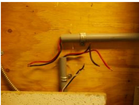
Figure 53: Exposed Wiring
