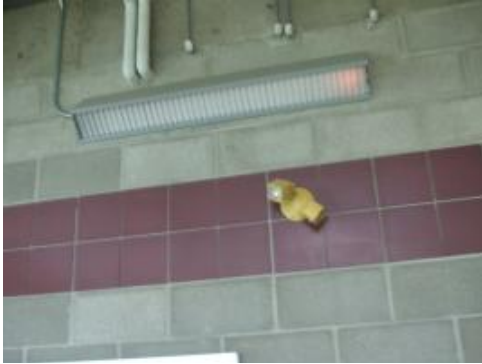
Figure 52: Trades and Technology Corridor Lighting
