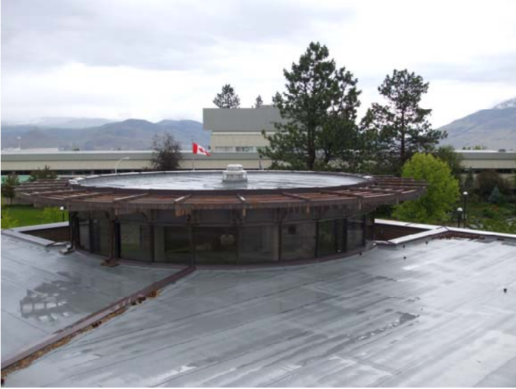
1. Attic Exhasut Fan.JPG
