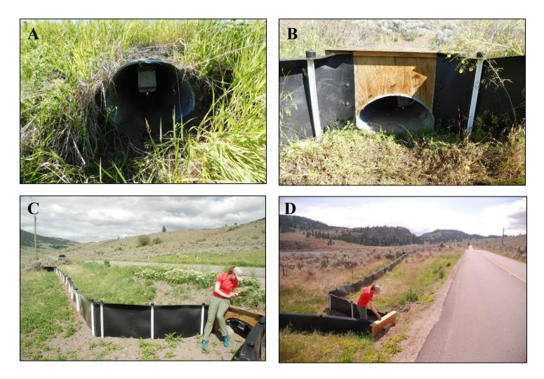
Figure 1.4. Examples of snake road mortality mitigation measures in the White Lake Basin, British Columbia, including A) a modified culvert equipped with a camera, with the entrance unaccompanied by fencing, B) a newly-installed semi-circular ecopassage equipped with a camera and fencing surrounding the entrance, and C & D) drift fencing positioned to funnel snakes into under-road ecopassages. (Photo credits: Karl Larsen)
